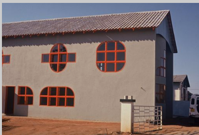
Fig 10. Chinese Agricultural Mission. 1992: The Author. Using lightweight fibre reinforced concrete roof tiles and concrete window frames was an attempt to foster local rural women's economic development.
